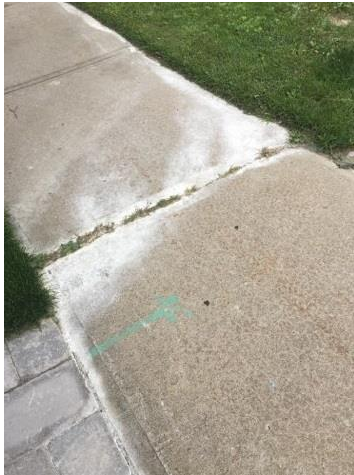
Figure 2 - Calcium residue left on driveway and sidewalk when using outside tap
